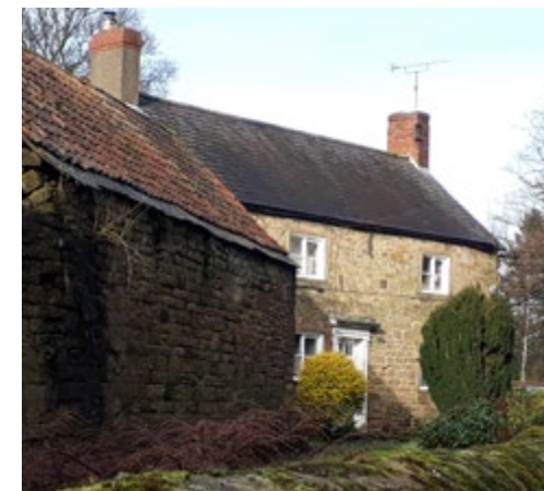
Traditional windows and doorcase, Stainsby
