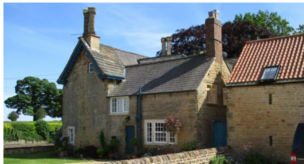
Oversailing eaves with barge boards, Hardwick and Rowthorne
